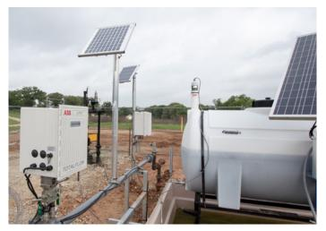
Fig. 1: Solar powered level application
